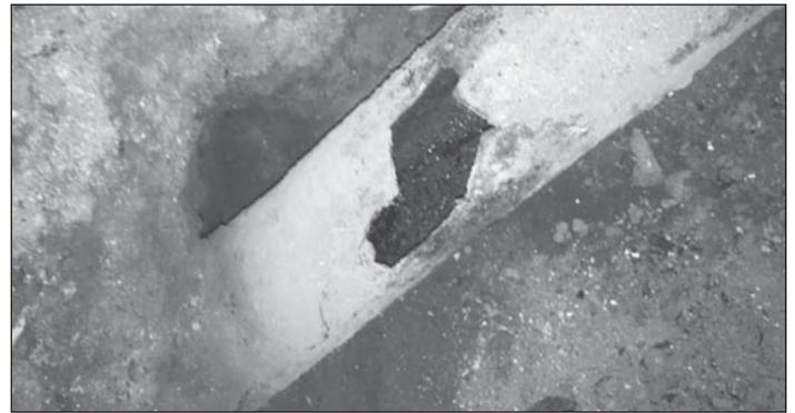
*Broken sanitary waste line to be excavated and replaced*
