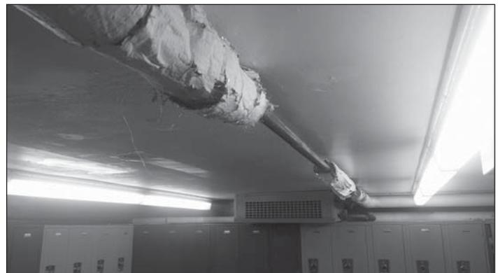
*Locker room plumbing insulation to be replaced*
