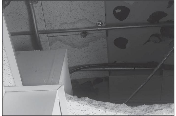
*Damaged ceilings caused by leaks in roof*
